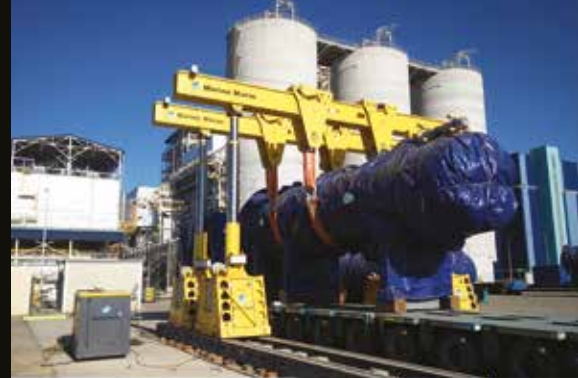
The Enerpac SL400 Gantry lifts the 138-ton high-pressure heater.
