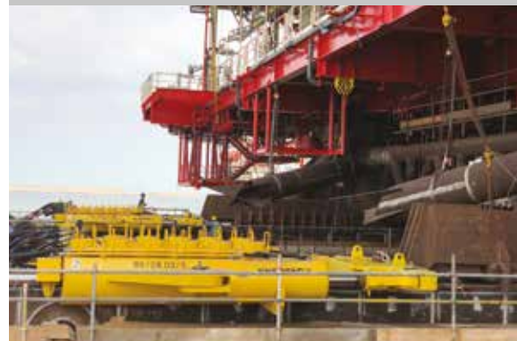
Enerpac 'Push-Pull' system for the platform module load-out.
