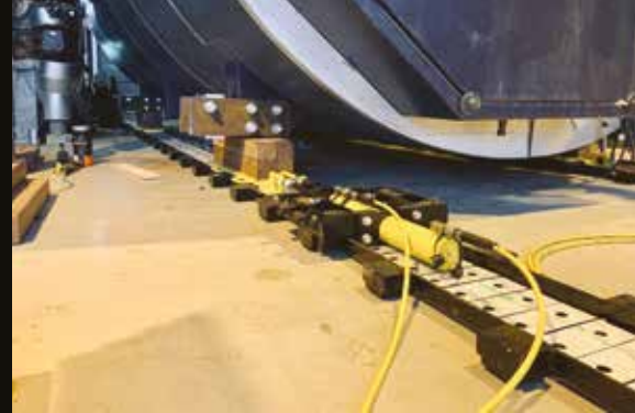
Preparing to skid the boiler out of the building.
