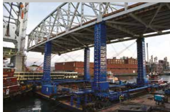
Positioning new bridge span into place.
