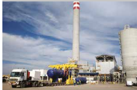
Delivering the high-pressure heater.
