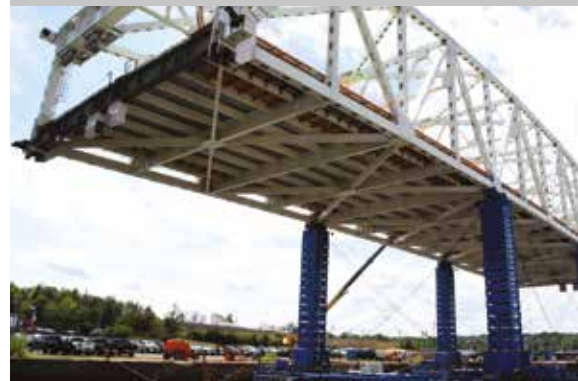
Fully lifted bridge ready for transport.
