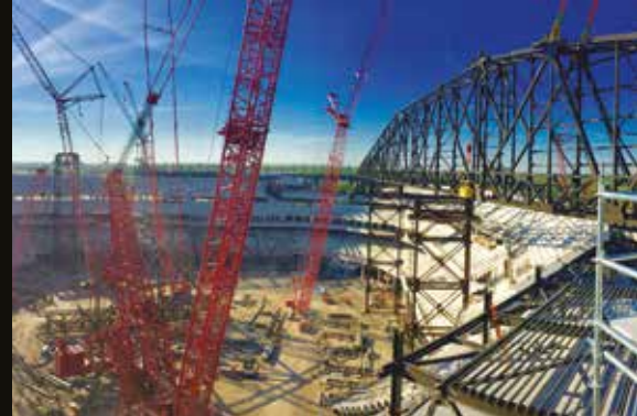
Enerpac SyncHoist system in use during roof truss picks.
