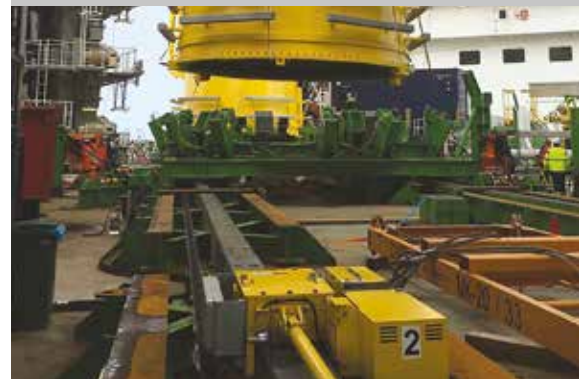
Loading of transition segments.
