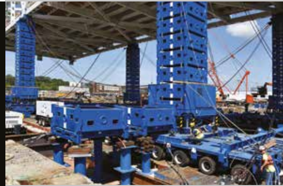
Beginning the lifting operations of new bridge from assembly site.
