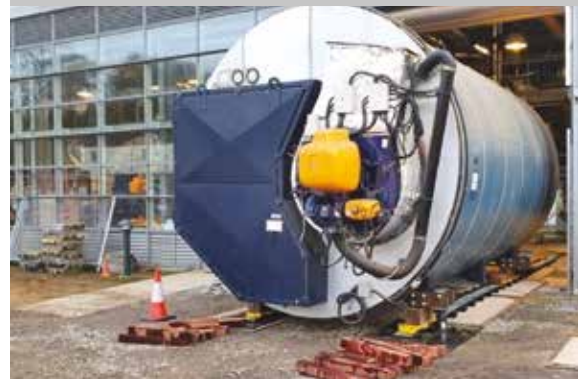
Boilers skidding in process.
