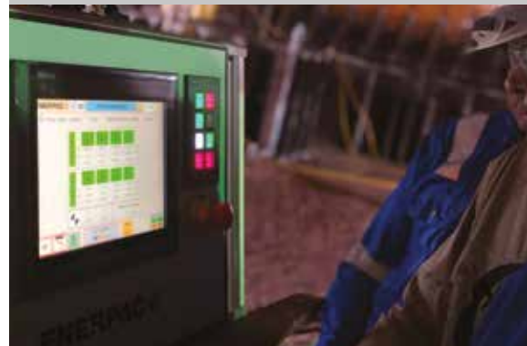
Effective control of the EVO system's network of 96 cylinders.
