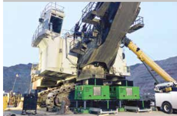
The Enerpac JS500 Jack-Up starts lifting operation.
